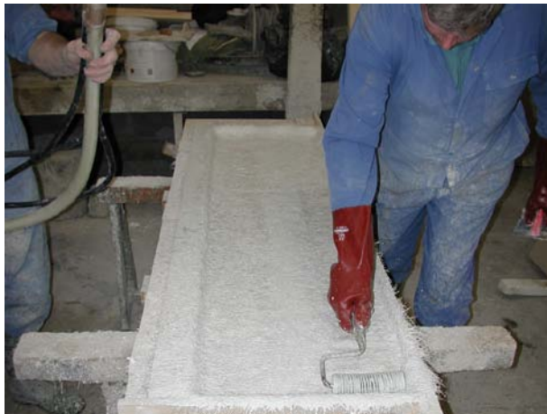
Figure 1.3 Compacting GRC using serrated roller
