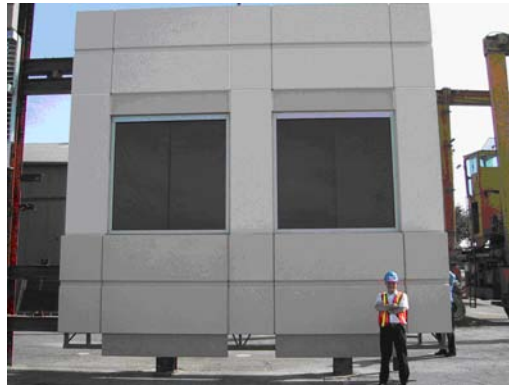
Figure 3.14 - Large Stud Frame Panel, USA
