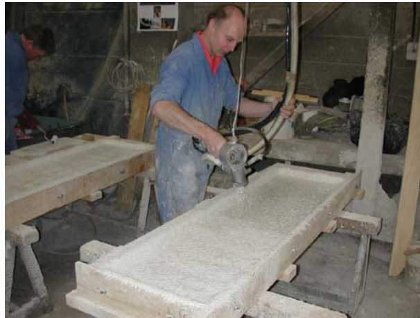
Figure 1.2 Spraying GRC into mould
