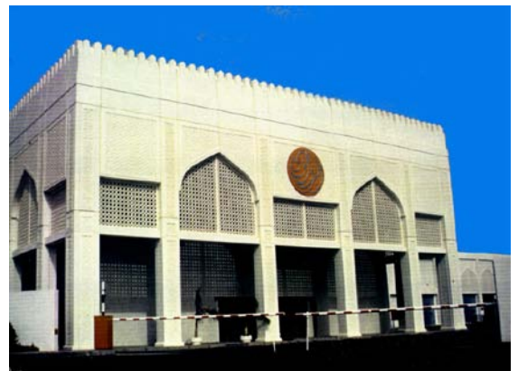
Figure 3.13 - Stud Frame Construction Car Showroom, Oman
