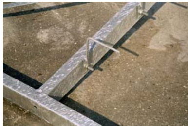
Figure 3.6 - Stud Frame fabricated from Rectangular Hollow Sections
