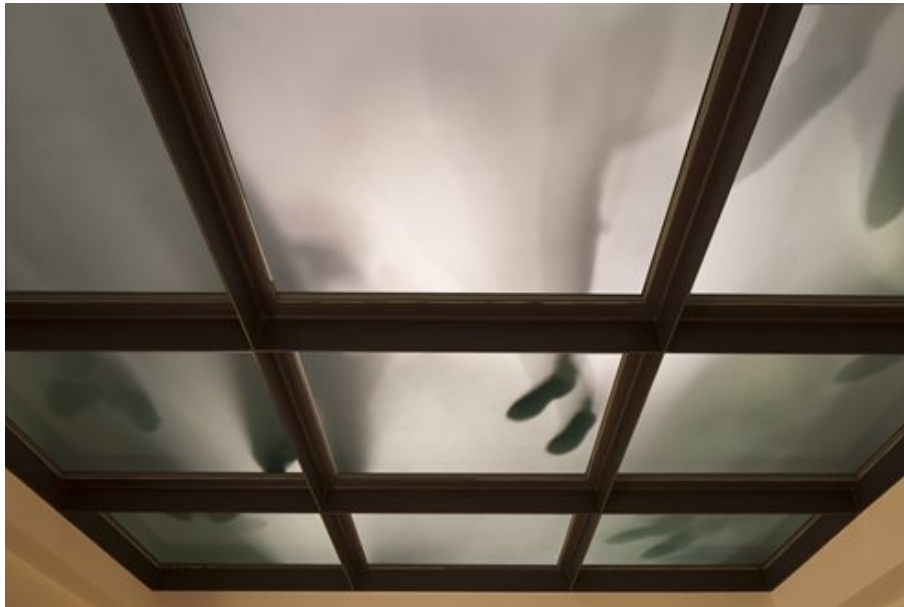
Sandblast coatings to face one of a walk-on rooflight provide a dual purpose with high anti-slip rating and privacy factor.
