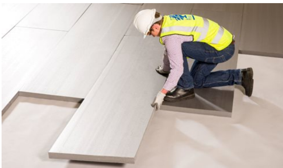
XPS insulation is not a hazardous substance or mixture. Nevertheless, appropriate PPE should be worn whilst handling and installing.
