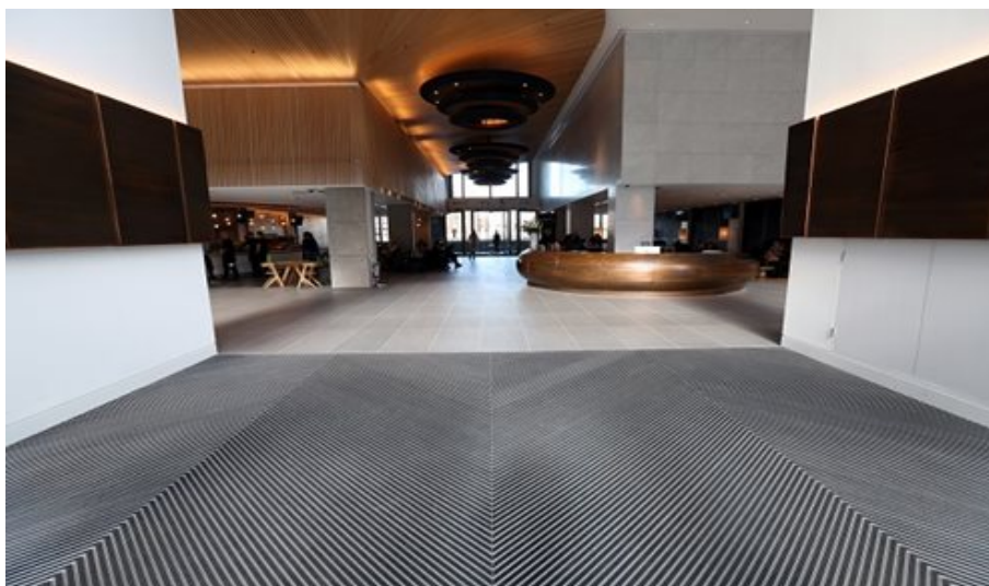
An appropriate Entrance Flooring System should be installed in commercial buildings and buildings used by general public to remove water and debris from foot and wheeled traffic.
