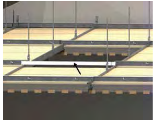
Step 4: Note that the cross bar is detached!
