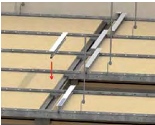
Step 5: Position it on the adjacent panel
