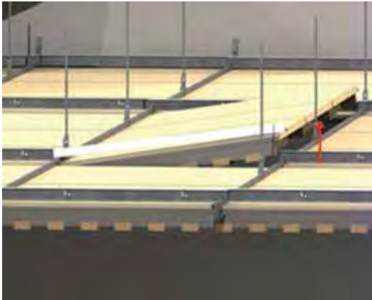
Step 1: Lift the panel
