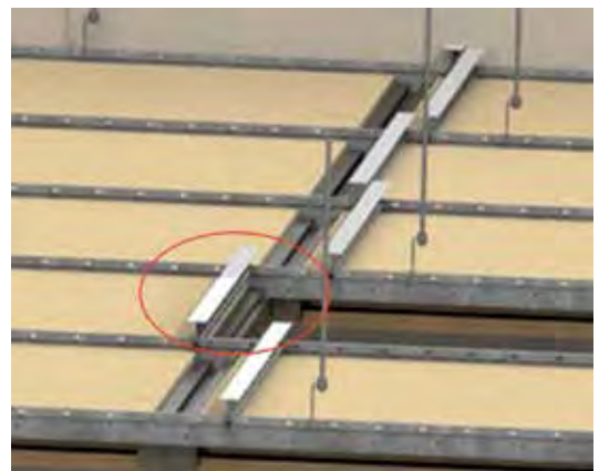
Step 6: Attach the cross bar above the adjacent panel
