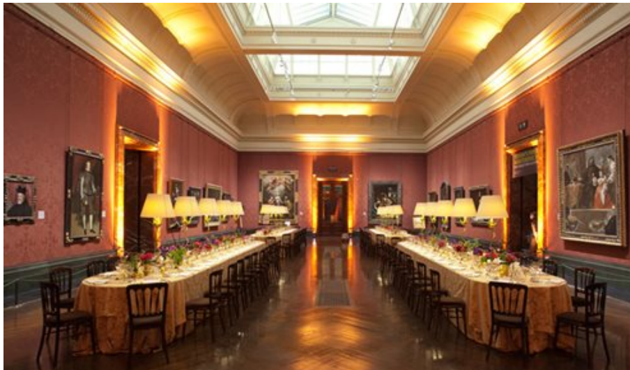
To minimise UV light transmission, diffused glazing with a satinovo white laminate was utilised, protecting the artwork below from solar glare.
