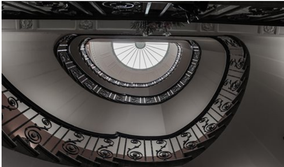
In most refurbishment projects, such as Somerset House, a bespoke rooflight design is the only feasible option, allowing replication of existing styles whilst achieving modern standards.
