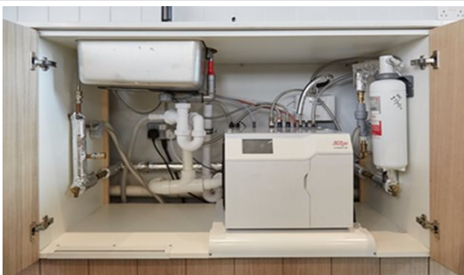
A twin chamber system is the most effective choice for a drinking water system as it saves energy and reduces water wastage.
