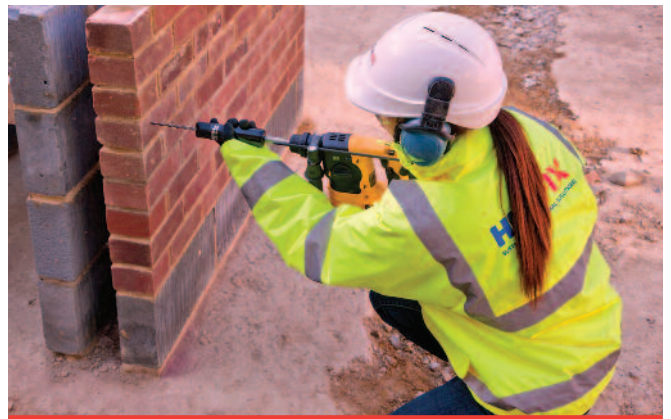
DryFix tie being power-driven into pilot hole
