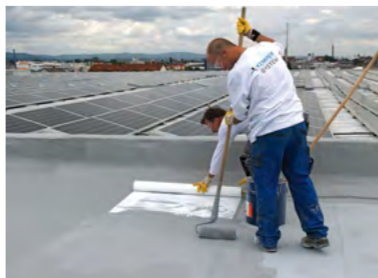
The roofing team applies the KEMPEROL® waterproofing membrane
