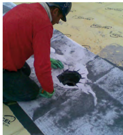
The drain outlet is fully incorporated into the seamless, cold applied, liquid waterproofing membrane.
