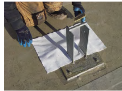
Installation of the waterproofing membrane.
