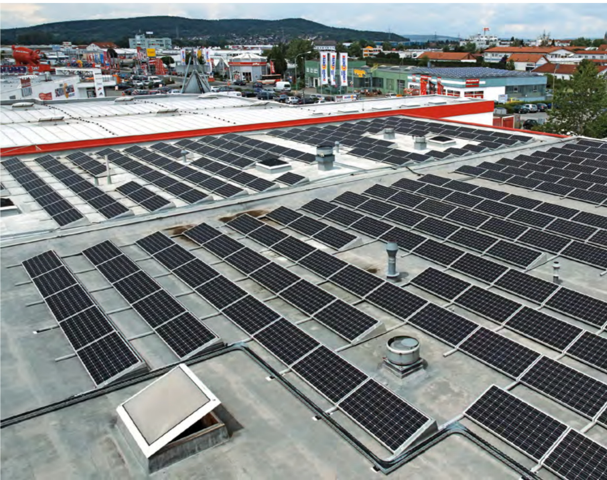
Some 10,000 m 2 of flat roof surfaces were rewaterproofed with KEMPEROL® liquid waterproofing before installing a photovoltaic system with an output of 406 kWp.
