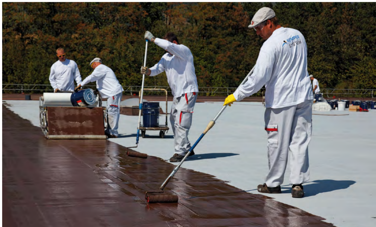
The KEMPERATOR enables large areas to be waterproofed quickly and easily.
