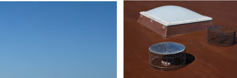
All details such as rooflights, roof outlets, junctions, joints and penetrations are incorporated seamlessly into the waterproofing on the surface.
