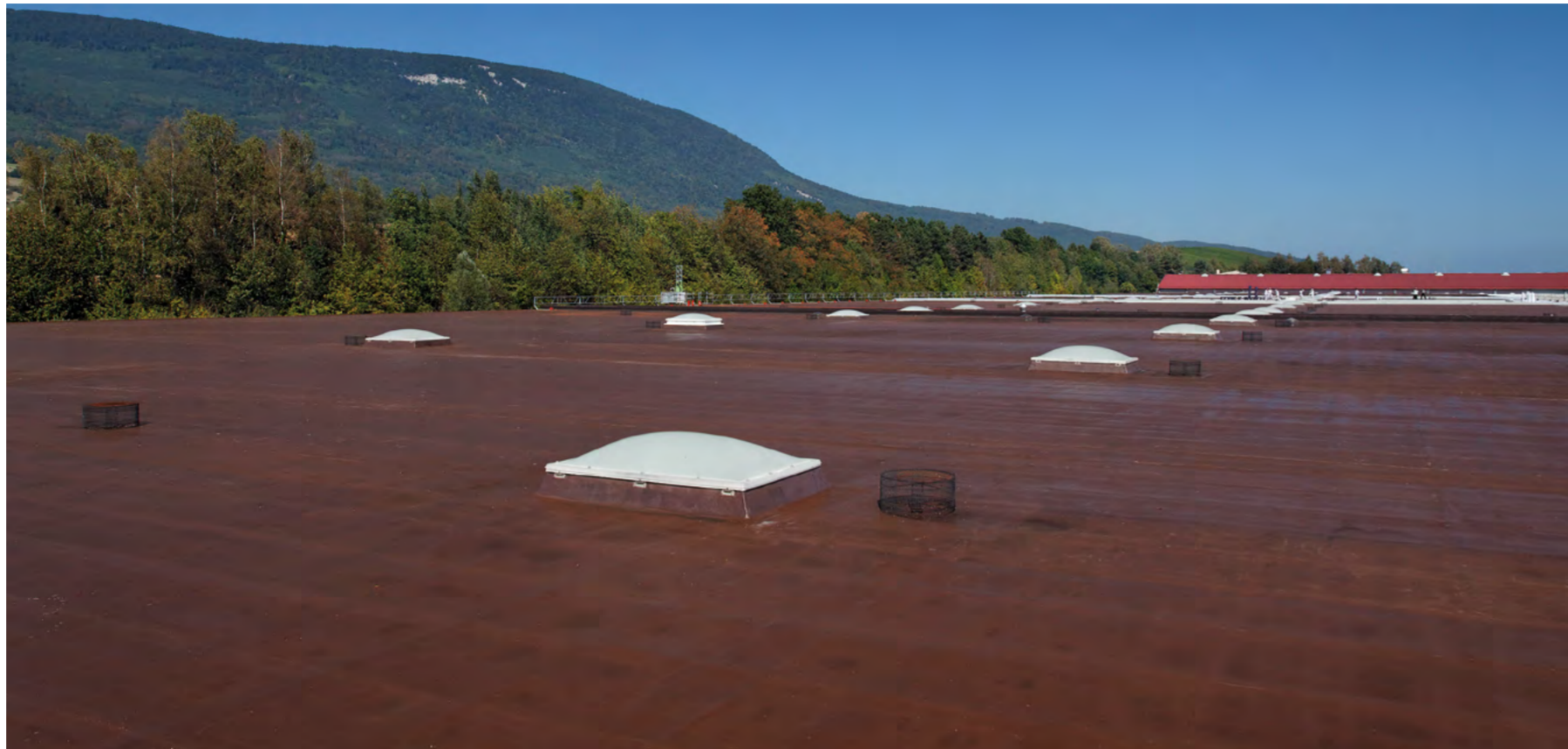
A total of 60 000 m² of flat roofs were waterproofed with KEMPEROL® V 210 at the Philip Morris plant.
