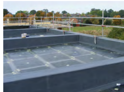
The flat roofs were waterproofed with KEMPEROL® as part of the complete Stratex Warm Roof System
