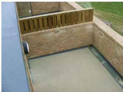
The balconies were waterproofed with KEMPEROL® and finished with KEMPERDUR® TC and KEMPERDUR® Coloured Quartz.
