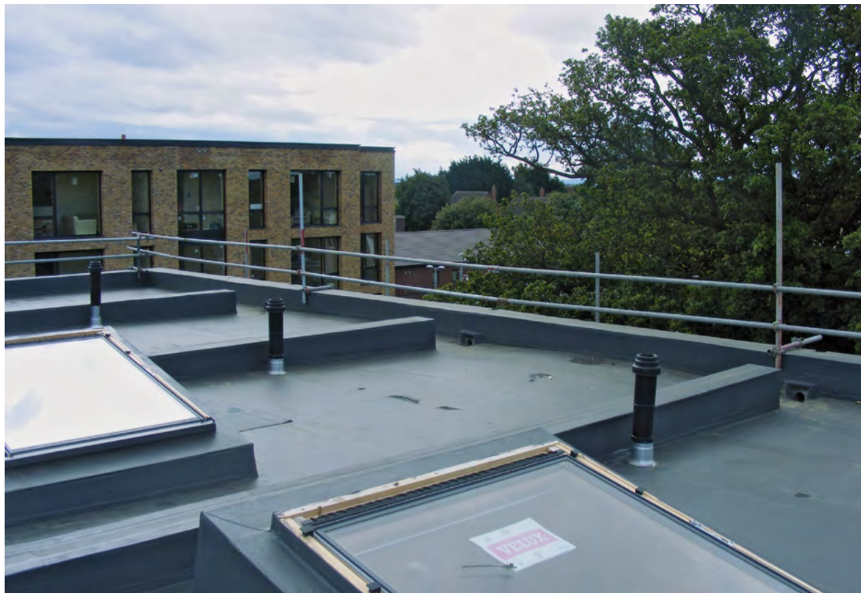
Customized work: all drains, pipes and upstands were seamlessly incorporated in the waterproofing membrane.
