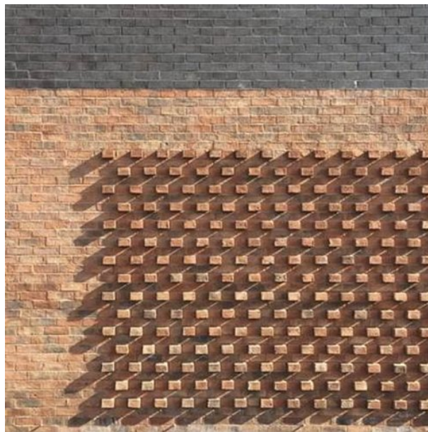
Projecting headers. Foundry, Salford. Architects: Sixtwo Architects
