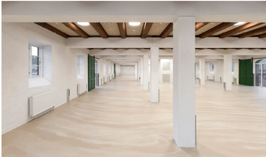
Resin comfort flooring installed in a commercial situation subject to busy use
