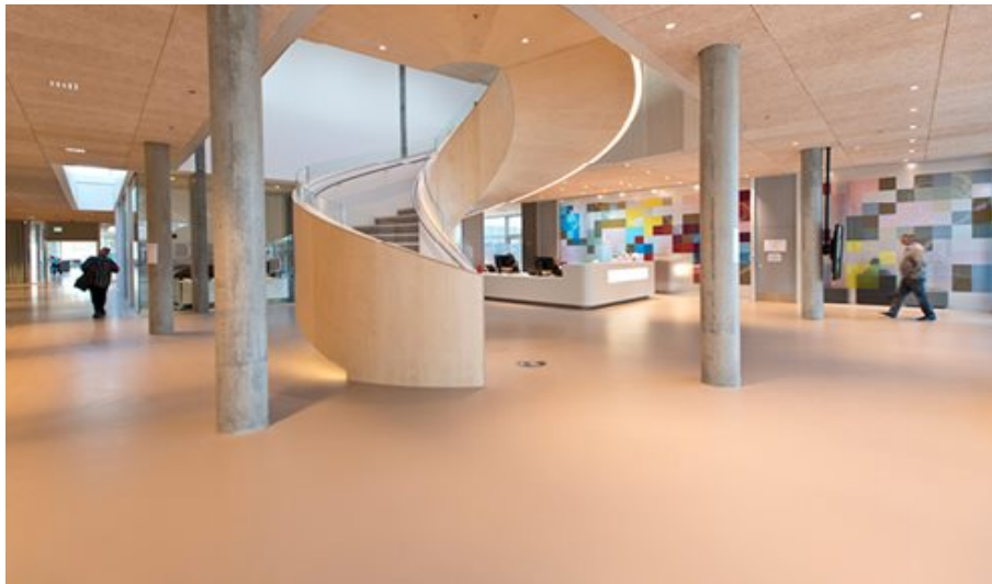
Resin comfort flooring installed in a hospital for durability and sound reducing performance
