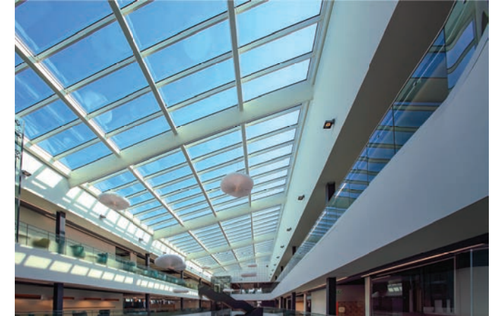
Prospero Business Park, Coventry Pendock Linea Atrium Beam Casings
