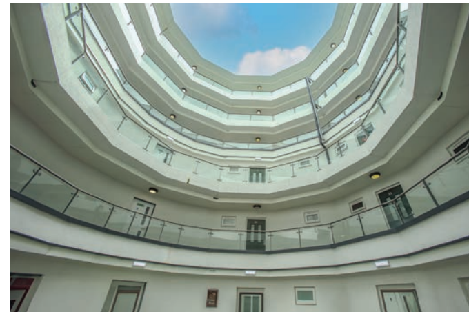
Phoenix Point, Thamesmead Pendock Profiles Metal Pipe Boxing
