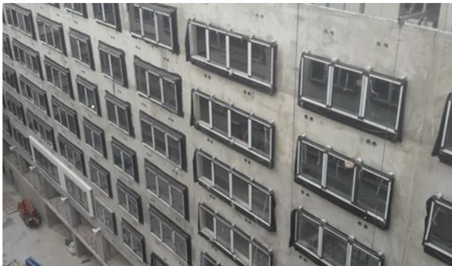
EPDM Membrane applied between window and concrete wall
