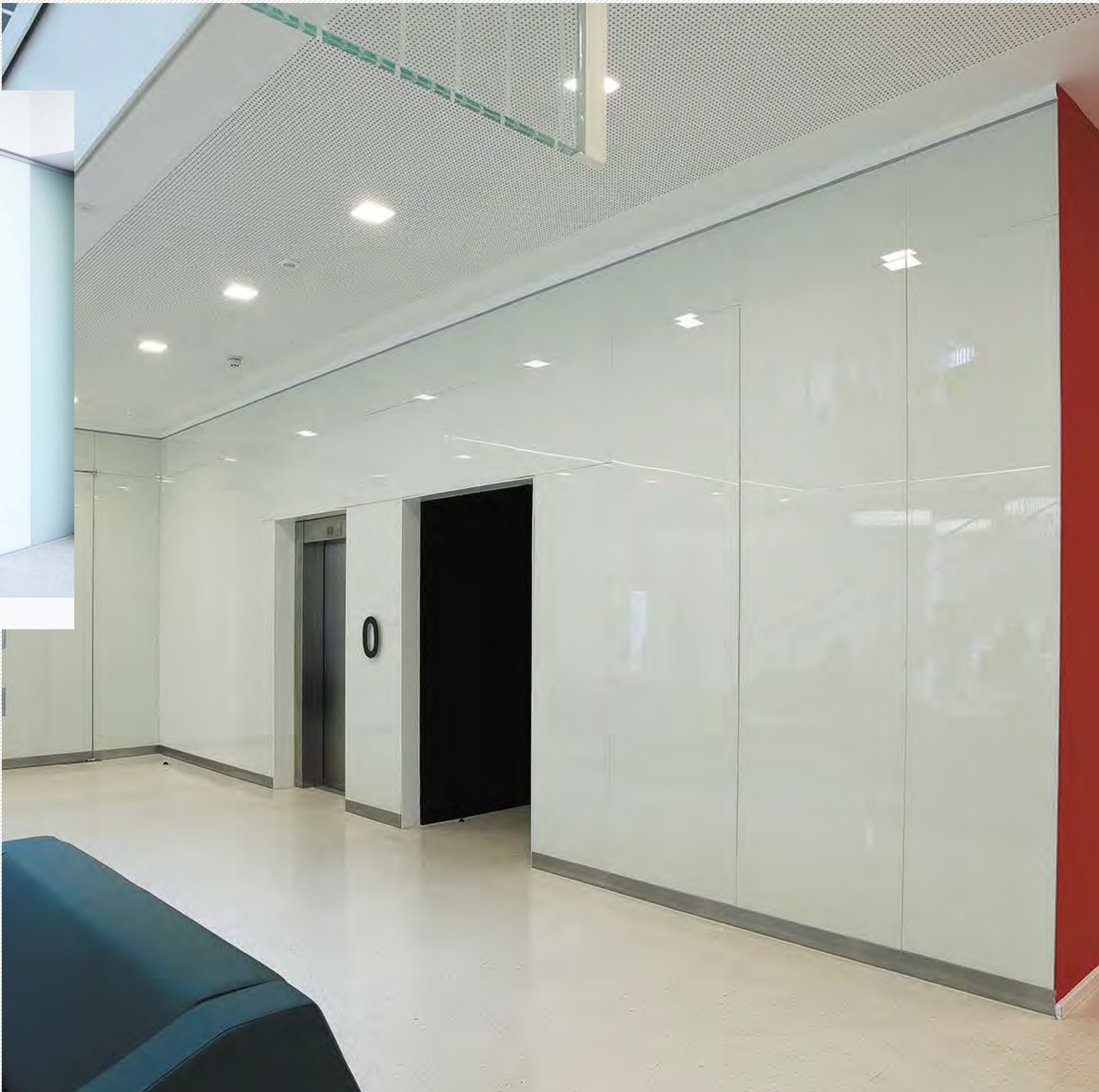
> Glass wall cladding in a lift lobby area
