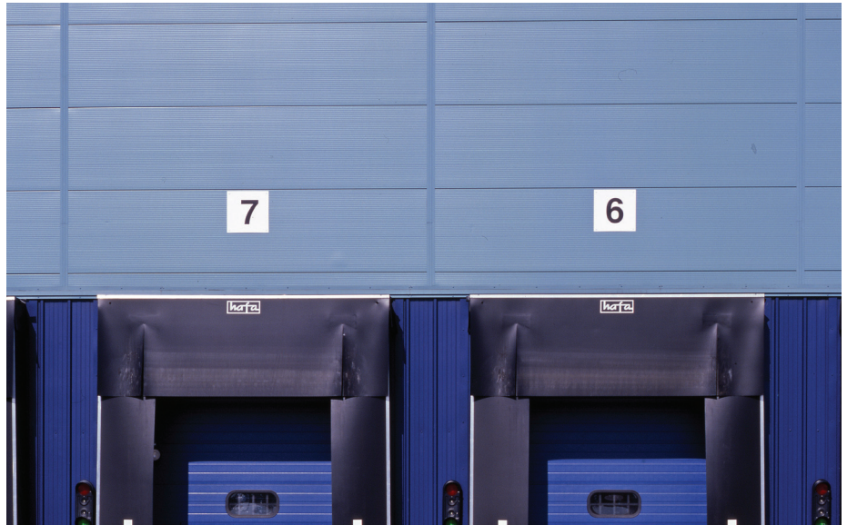
Vertical breaks incorporated into horizontal cladding.
