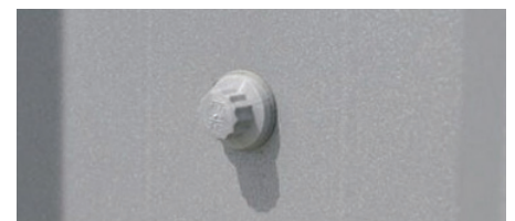
Correctly tightened colour-matched fastening.
