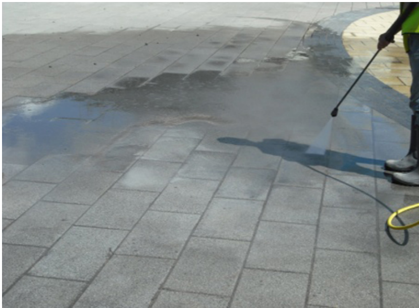
Image shows the surplus 'wash off' stage of the slurry method.
