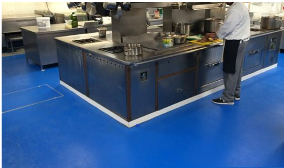
Polyurethane floor screed installed in a commercial kitchen
