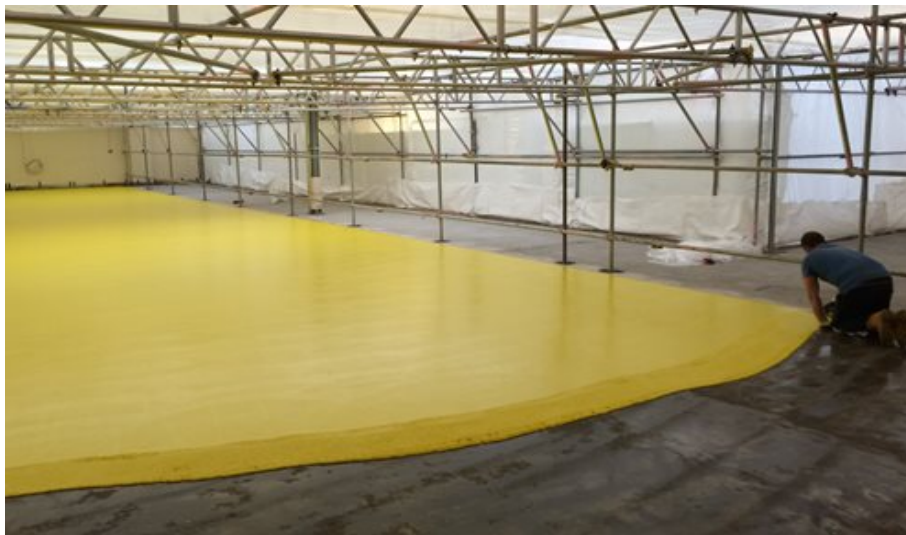
Polyurethane floor screed being installed onto prepared and primed concrete
