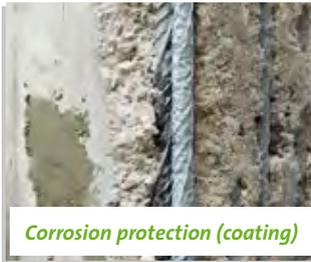
Corrosion protection (coating)
