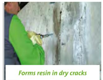
Forms resin in dry cracks
