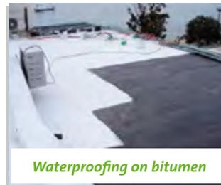
Waterproofing on bitumen
