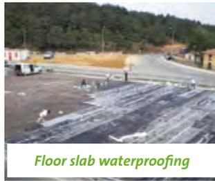
Floor slab waterproofing
