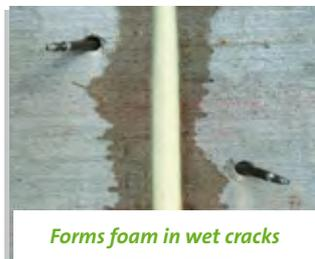
Forms foam in wet cracks
