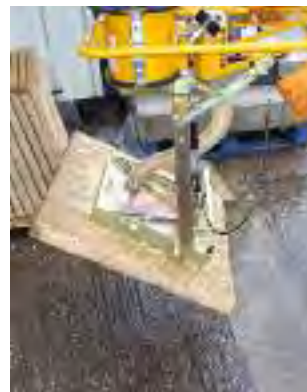
Sequence shows vertically stacked flags brought to horizontal position using vacuum lifting machinery
