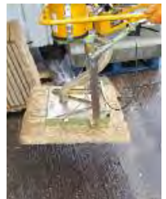
Sequence shows vertically stacked flags brought to horizontal position using vacuum lifting machinery
