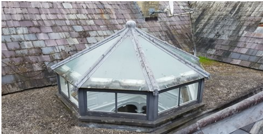
Rooflight styles from the early 1800's featured a mixture of timber and metal constructions and wire cast glazing.
