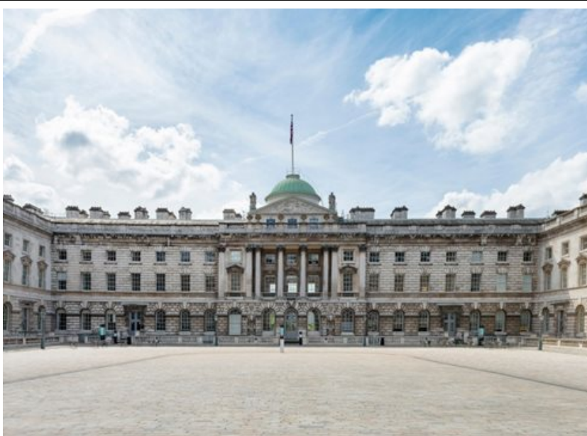
Somerset House was built in the neo-classical architectural style and has a very distinct designs of rooflights.
