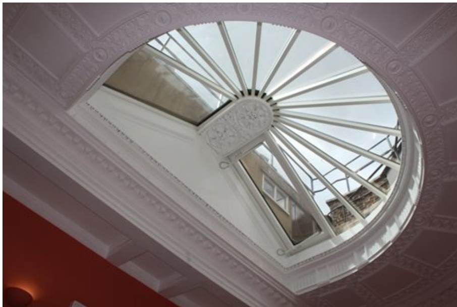
Bespoke Ogee heritage glazing bar developed specifically to match existing profile. Existing design features retained with modern performance values.
