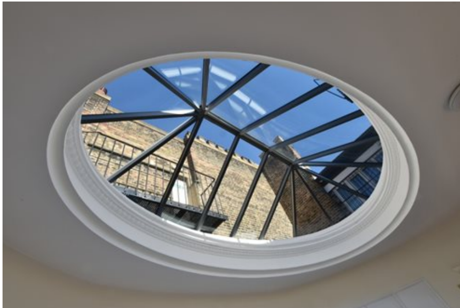
Modern rooflight designed with minimal glazing bars, junctions and ridge detail to closely match original Victorian cast iron crittal style rooflights.
