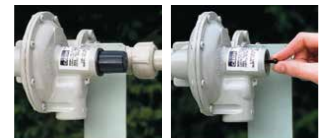
Resetting the tank regulator
