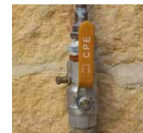
Step 2 B. Emergency control valve - Open valve
